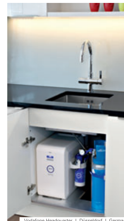
Vodafone Headquarter | Düsseldorf | Germany
